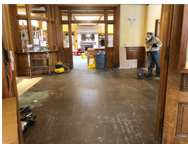
The main floor carpeting gets replaced.
