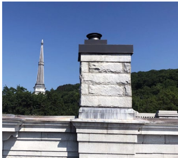
The freshly recapped library chimney, part of the GLL renovations.
